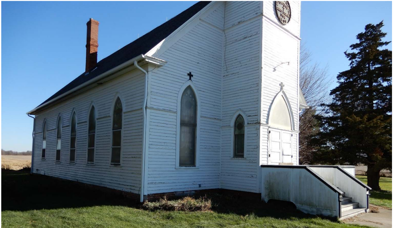
Looking NE at St. Malachy's. Photo taken 11/13/2020.
