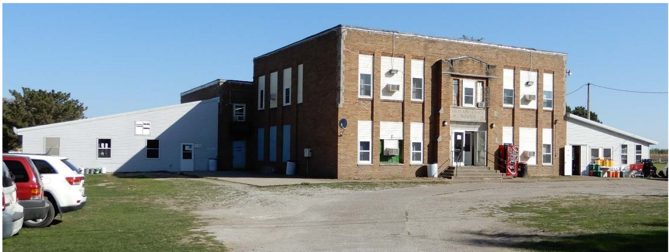
2020 Photograph of the Conesville School built in 1934. Looking ESE. Photograph taken October 7, 2020.
