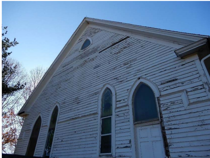
Detail of rear gable end of St. Malachy's. Photo taken 11/13/2020.
