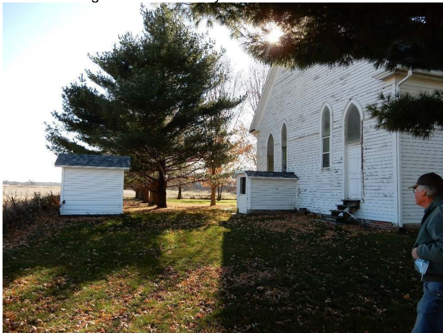
Looking at rear of St. Malachy's with later privy to left of building and cellar entry projecting out from rear of building. Photo taken 11/13/2020.
