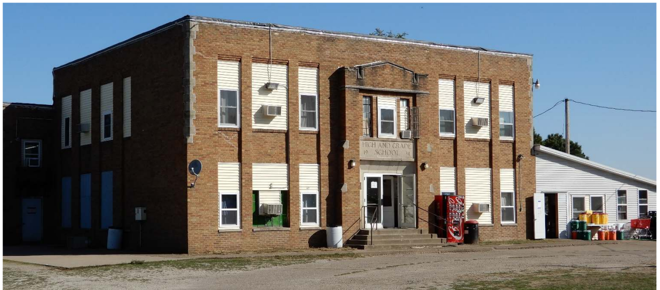
2020 photograph of the Conesville School looking ESE. Photograph taken October 7, 2020.
