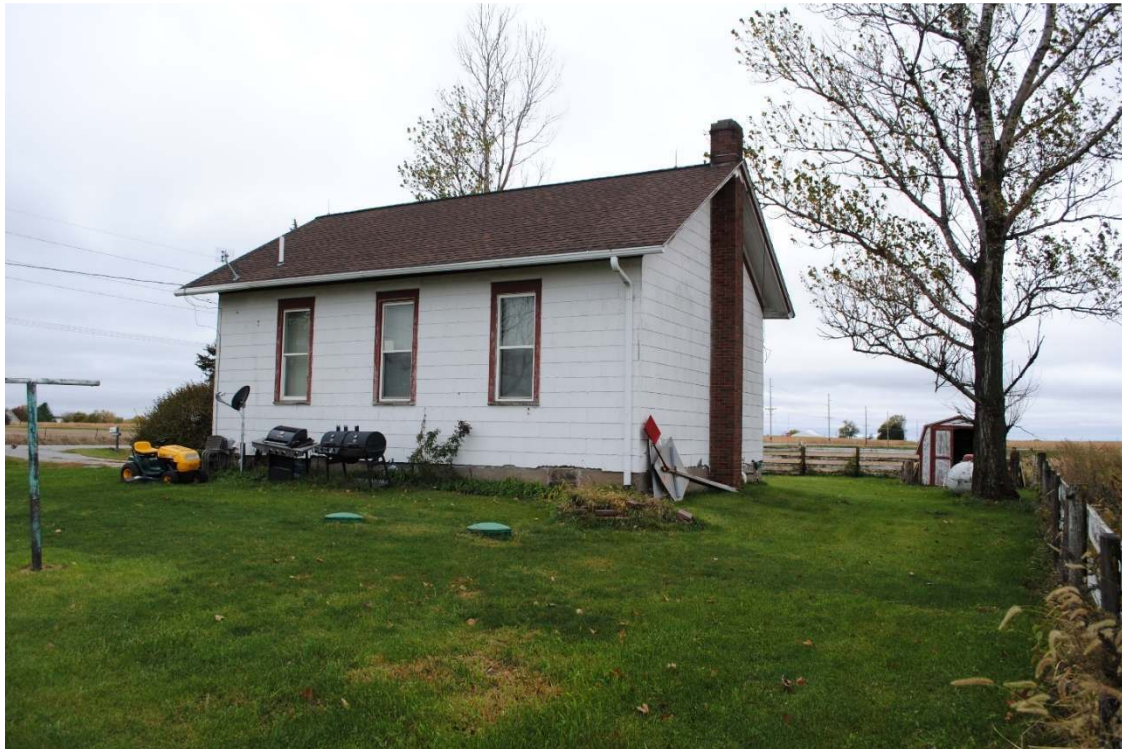
East and north sides of school. Facing southwest. Photo taken in 2020.
