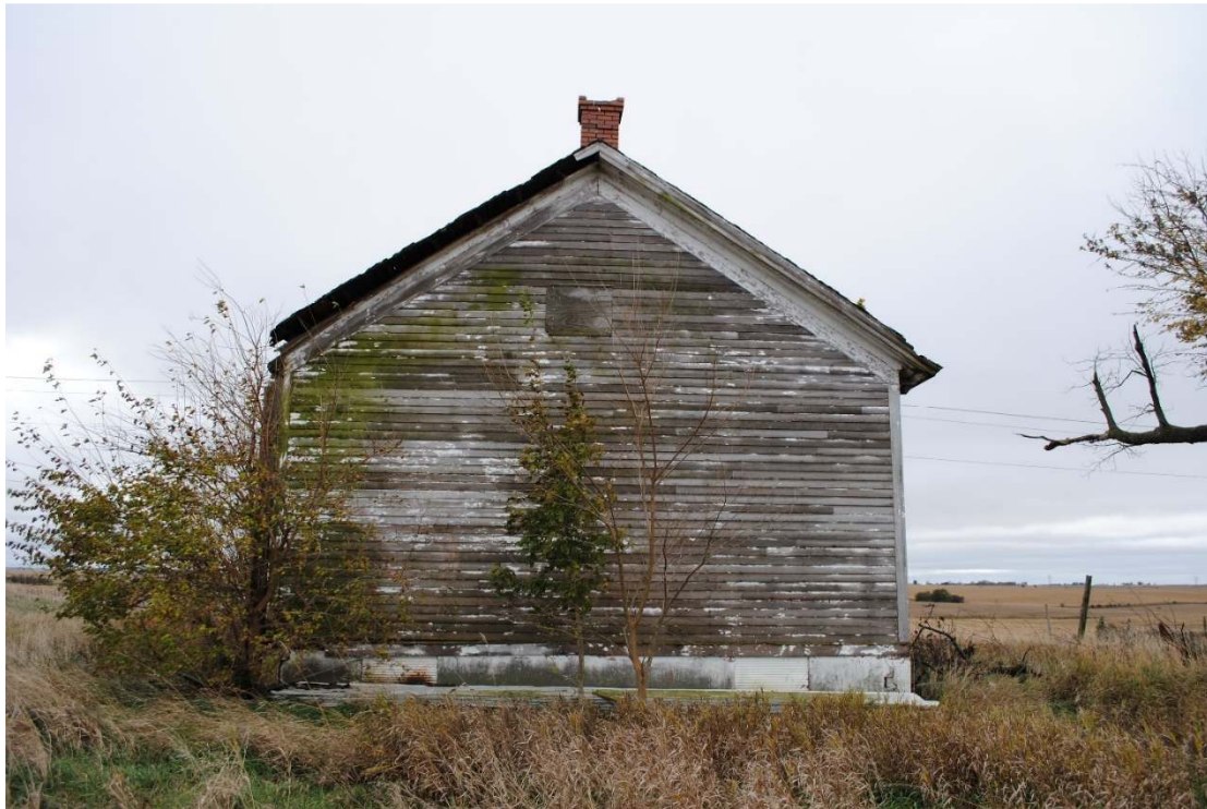
Prospect Hill School #3. Facing south.
