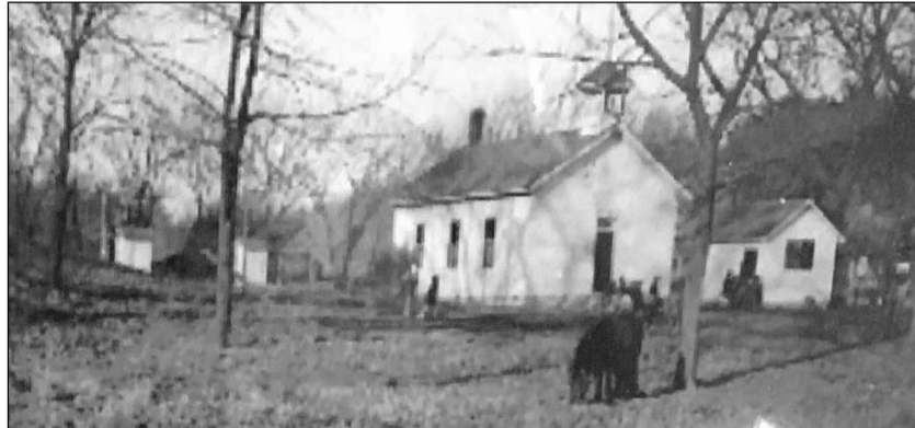
Figure 300. Circa 1936 photograph of the Green Valley Schoolhouse and its outbuildings. Source: Notebook at Melpine Schoolhouse, Wildcat Den State Park.
