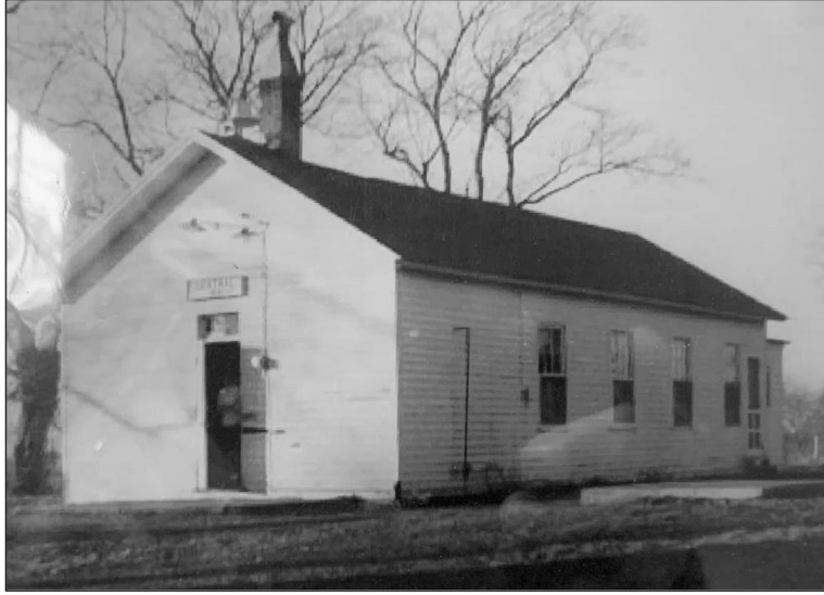
Figure 297. Undated photograph of the Central Schoolhouse. Source: Photograph display at Melpine School, Wildcat Den State Park.
