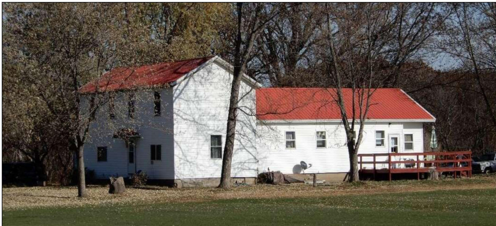
Figure 299. Rear section of this house at 2469 Cranston Road in Cedar Township is the former Central #4 Schoolhouse. Photo taken November 6, 2020.
