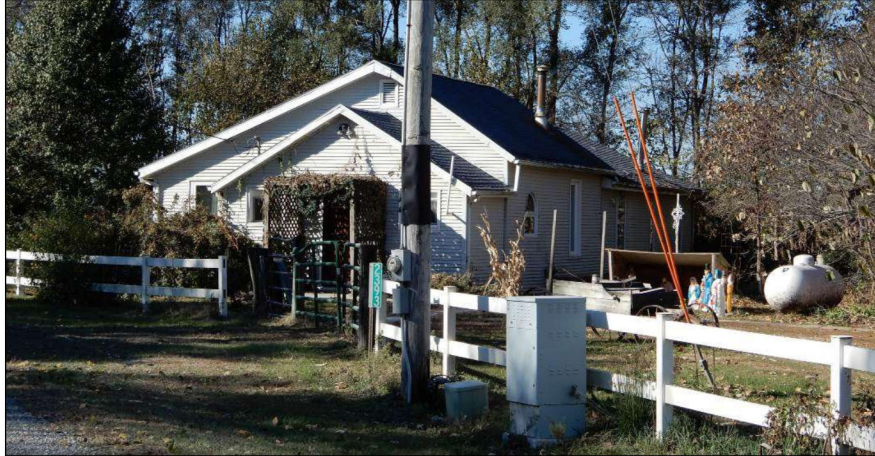
Figure 317. Mittman School at 2393 Mittman Rd where it was remodeled into a residence. Photo taken October 31, 2020
