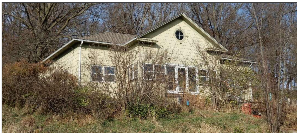
Figure 178. Former Fairport Schoolhouse at 3385 Pearl Avenue in 2020 showing additional modifications to the front-gabled façade. Photograph taken November 19, 2020.
