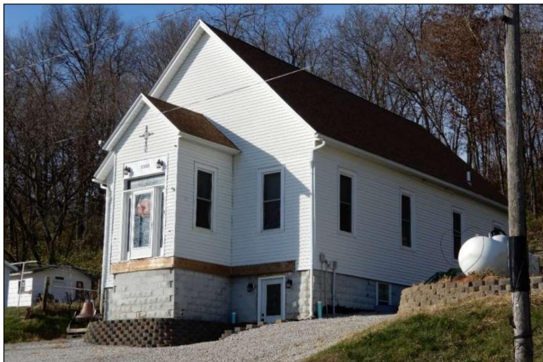
Figure 202. Former Fairport Church, now a house at 3383 Pearl Ave, with modern foundation and stairs removed. Photo taken November 19, 2020.
