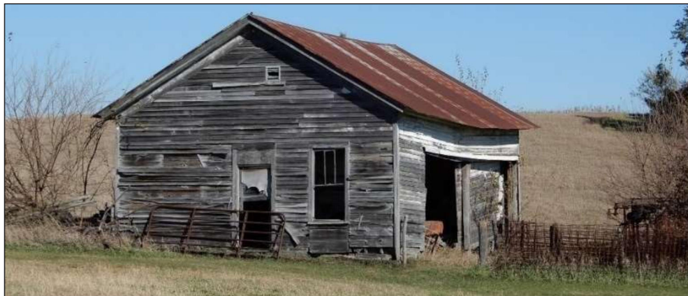
Figure 207. Fairview Schoolhouse at its moved location (70-01778). Photo taken October 31, 2020
