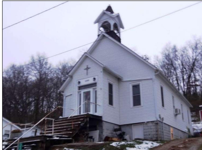
Figure 201. Photograph of Fairport Church in 2016.
