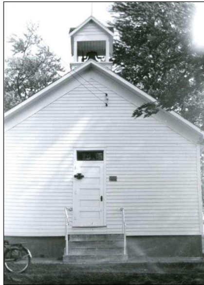
Figure 104. Circa 1947 photograph of the Yankee Hallow School. Copy provided by Muscatine County HPC.
