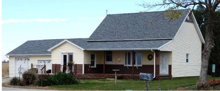
Figure 65. Former Independence Schoolhouse at 1572 Iron City Avenue in October 2020.
