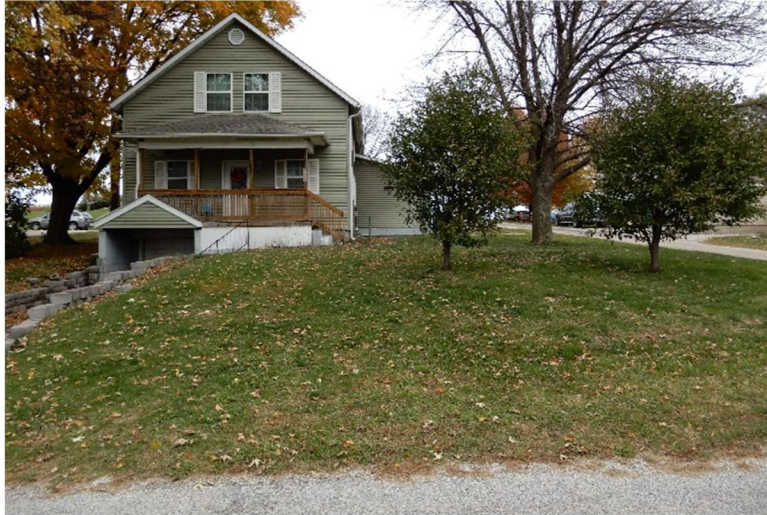
Figure 72. Site of former Adventist Church (non-extant) now the location of a house at 311 5th Street in Atalissa. Photo taken October 27, 2020.
