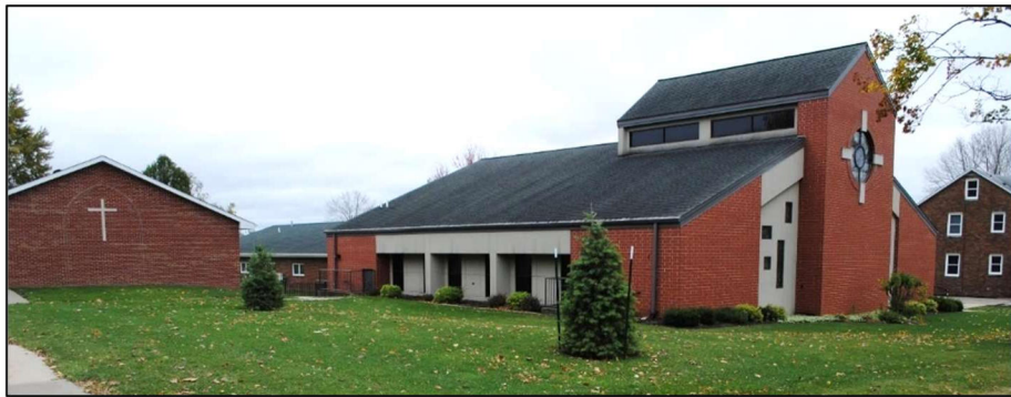
Figure 134. Extant St. Mary's Catholic Church in 2020.
