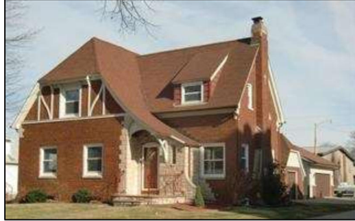
Figure 137. 1948 parsonage for the Zion Lutheran Church and located next to the church. Source: Assessor's photograph (Beacon).
