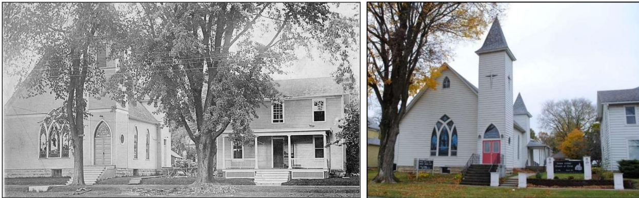
Figure 131. Grace Reformed Church and Manse circa 1910 (left) and Grace United Church of Christ in 2020 (right). Historical photograph provided by Muscatine County HPC.
