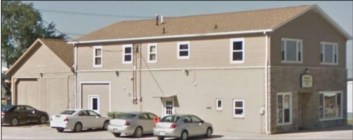
Figure 106. Former Yankee Hollow Schoolhouse attached to the rear of the Brammeier Chiropractic Office at 109 5th Street in Durant.
