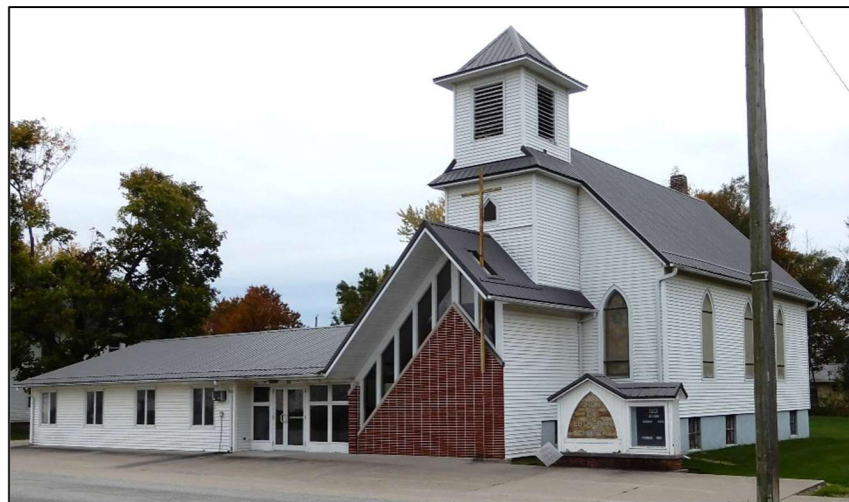
Figure 74. Zion Evangelical Lutheran Church in October 2020.
