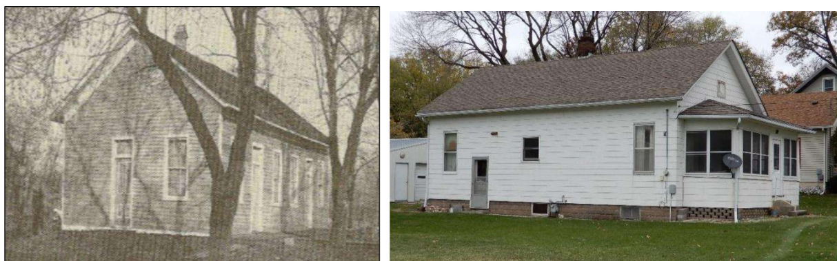
Figure 36. Friends Meeting House in West Liberty pre-1915 (left) and Friends Meeting House today at 803 N. Columbus St (right). Source: Hise ed. 1938; Photo taken October 27, 2020.
