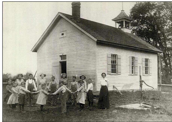
Figure 17. Circa 1900 photograph of Federal Hill School. Photograph provided by Jim Birkett.
