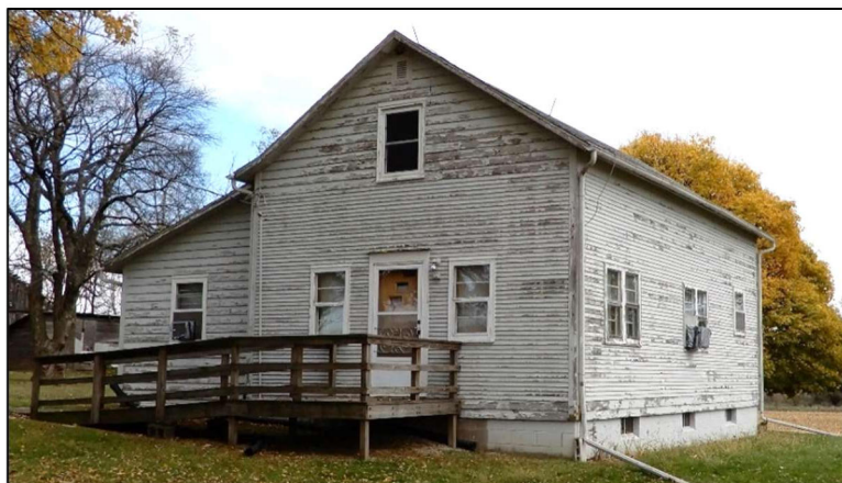
Figure 55. Former Union Valley Schoolhouse, moved and made into a residence at 1873 Highway 6. Photo taken October 27, 2020.
